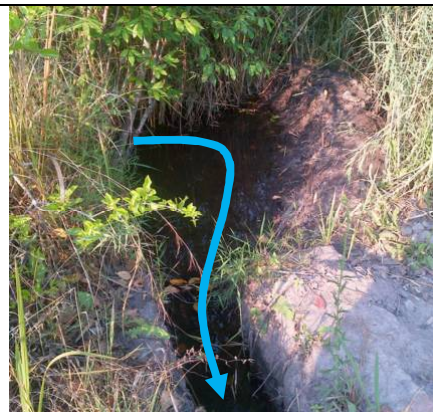
The fish farm is supplied with water by damming a small perennial stream with an earth dam, which has to be rebuilt after the rainy season.
