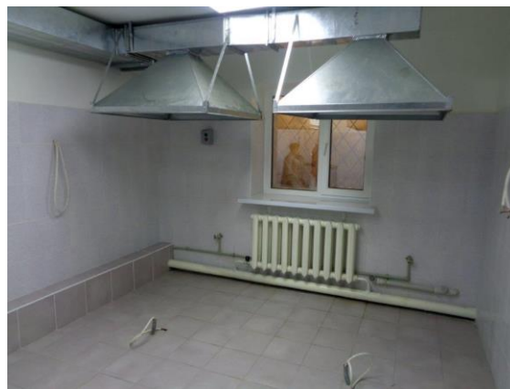
Photo 6: A future autoclaving room with the ventilation hoods in place.
