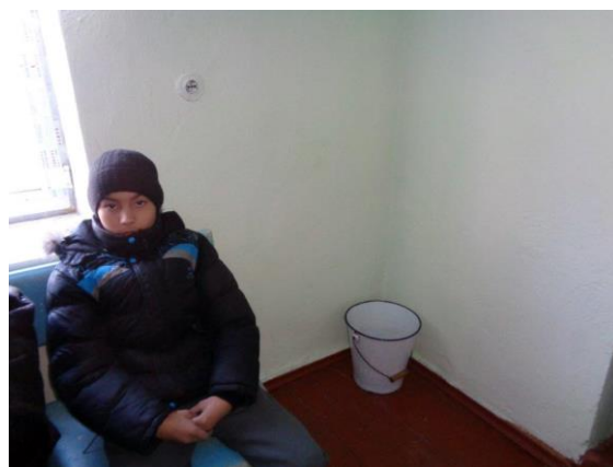
Photo 8: In the Besh-Kyungei Village FAP the autoclave is to be installed in the tiny waiting room where the bucket is. This is not an ideal solution and may require further work from the project to ensure that a satisfactory solution is found.
