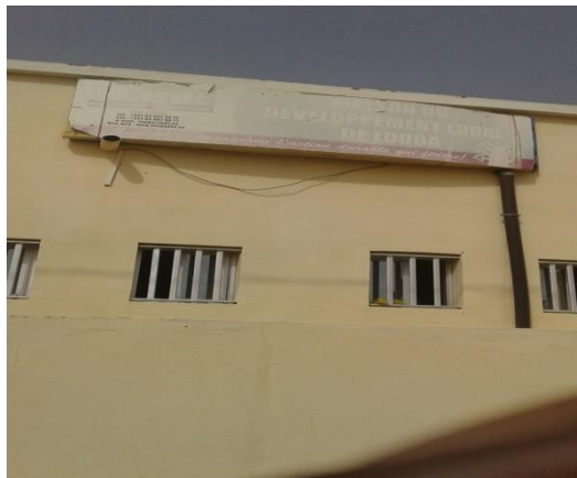
Figure 9: Facade of the Louga MDL currently occupied by the electoral registration commission
