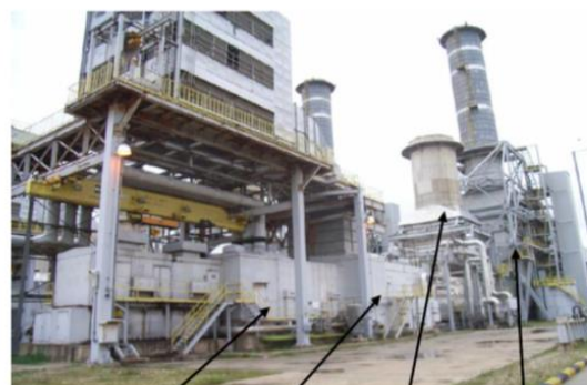
Unit 1 Generator, Gas Turbine, Exhaust Bypass Stack and Boiler
