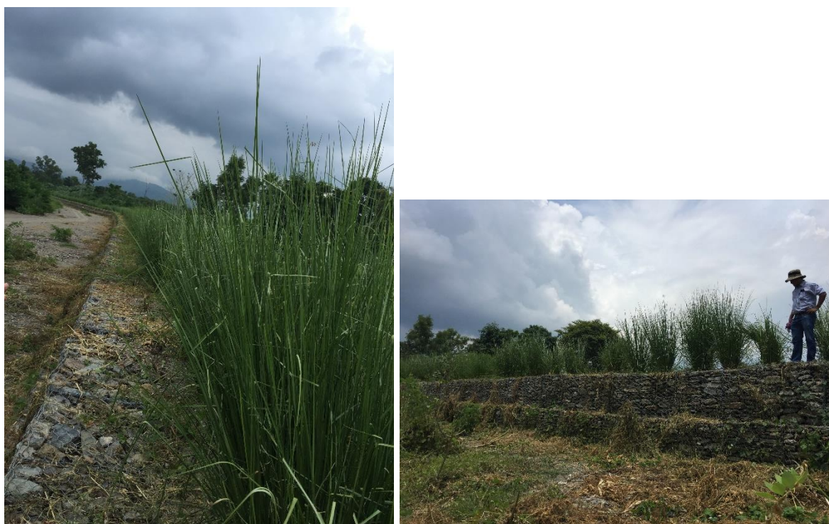
Figure 4-12: Earth flood defence with Vetiver grass planted and gabion basket protection on the river side
