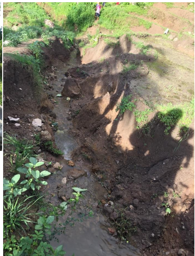
Figure 4-6: Rapidly eroding earthen channel
