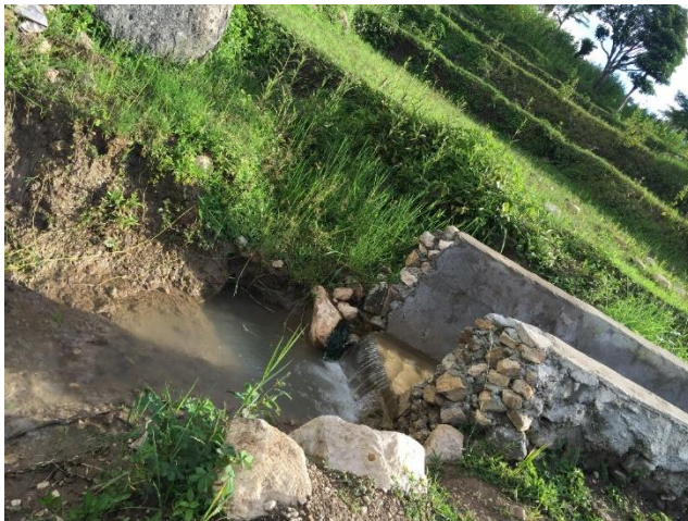
Figure 4-5: End of the irrigation channel outfalling to earthen channel. Eroded rice paddy on upslope just visible
