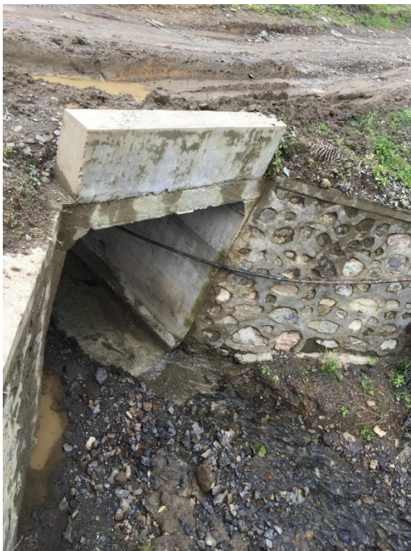
Figure 4-7: Wing wall and gabion baskets extending the protection on the upstream side of the bridge. Bio-engineering measures are also visible on the upstream banks
