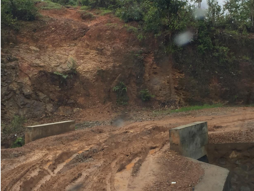
Figure 4-9: Heavily eroding road surface of one of the bridges. As the picture shows, there is ponding on the bridge which will lead to further erosion and exposure of the top of the bridge.
