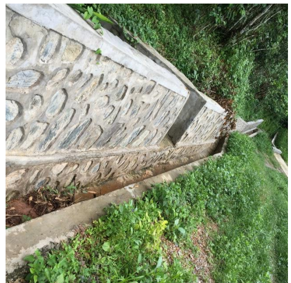
Figure 4-10: Drainage channel along the Maubalarisa road. Extensive vegetation of the slopes is also visible
