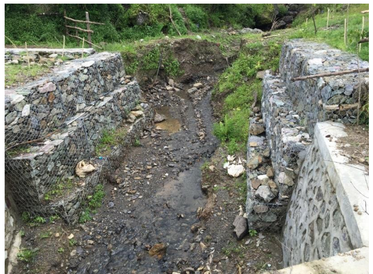
Figure 4-7: Wing wall and gabion baskets extending the protection on the upstream side of the bridge. Bio-engineering measures are also visible on the upstream banks
