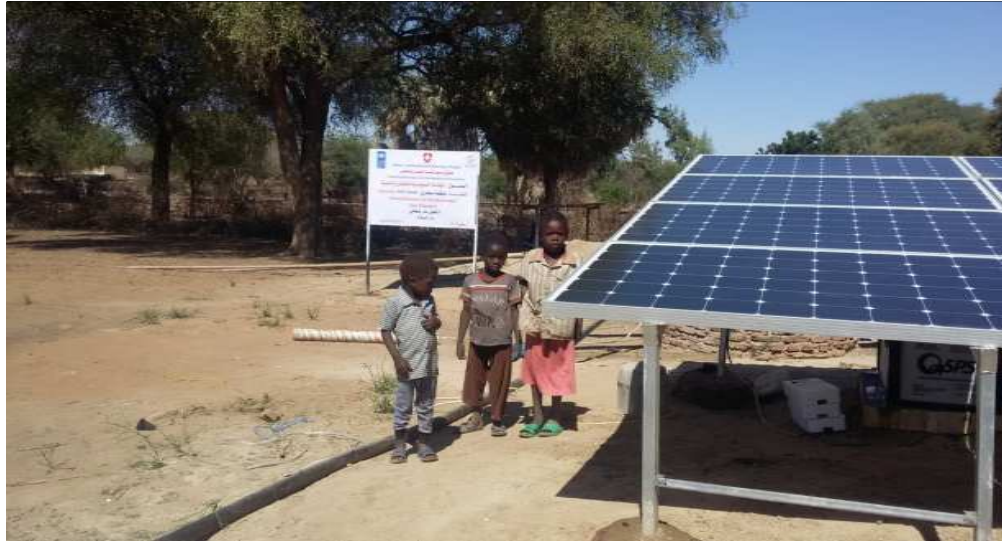
Solar Power pannel for pumping water - Darelsalam North Darfur
