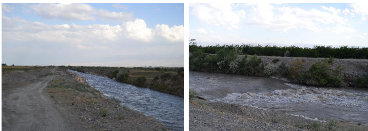
Absent (left) and present weirs at Zarafshan right bank canal (right)
