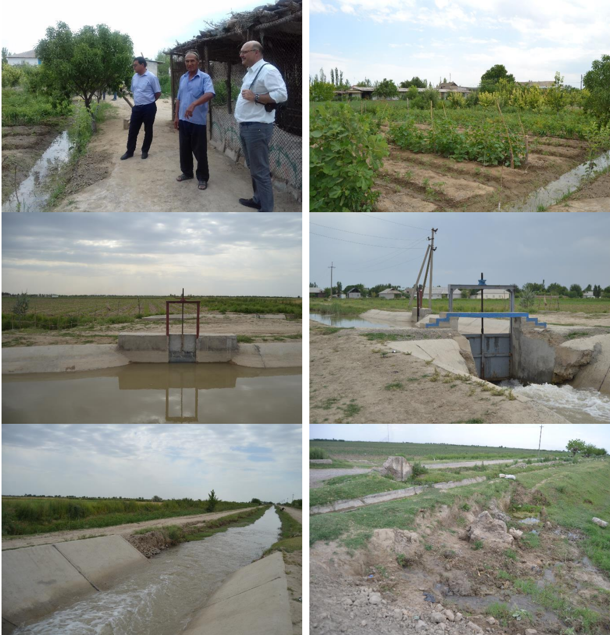
Field visit Lower-Syrdarya region: Visit of household irrigation pilot, Soyibobod village (top left & right); completed works of distribution structures at the Yuksalish canal (middle left & right); Bank erosion (left bank) after the end of lined canals (bottom left); uncontrolled seepage to the fields from small canals (bottom right).
