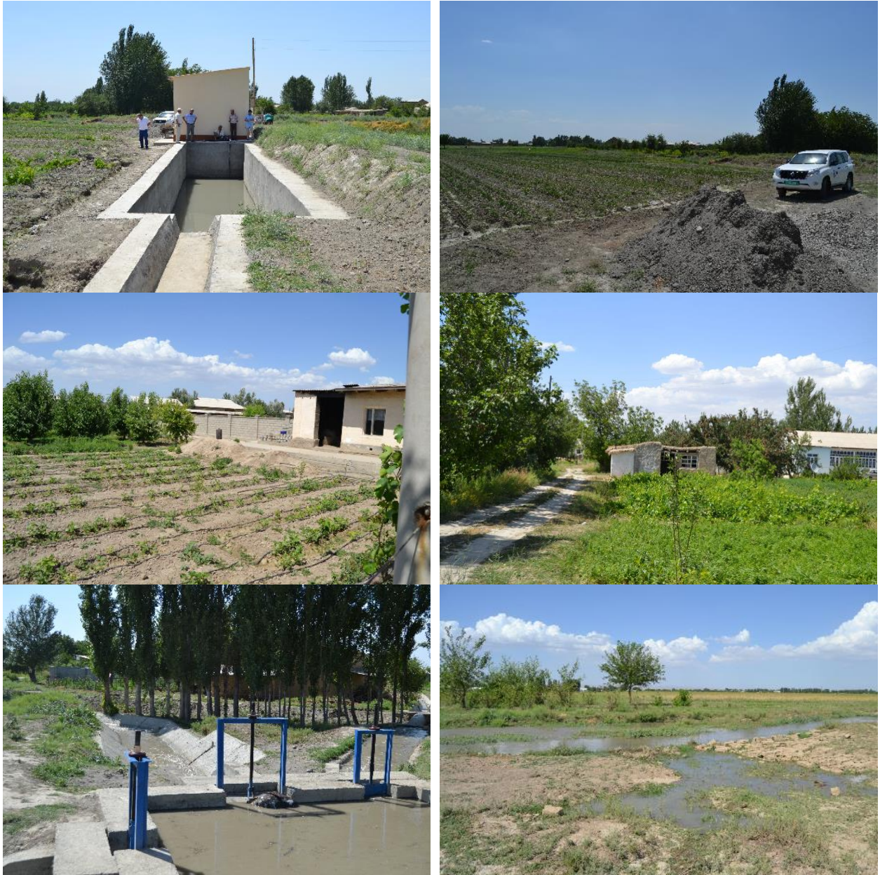
Field visit in the Zarafshan region: Pumping station, reservoir and tree and grape nursery at "Yangi Nav" farm (top left & right); Drip irrigation at household farm (2 nd row left); Favourable climate for vegetation and growth in the neighbouring village are (2 nd right); Blocked weir and uncontrolled seepage at Huja Buston canal (bottom left and right);
