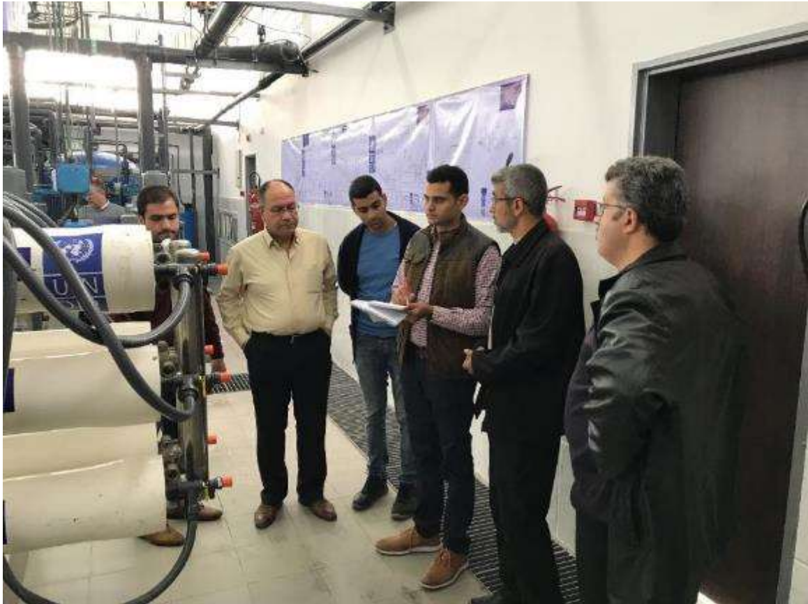
Fig. 11: Field Audit Team Evaluating the Rehabilitated Desalination Unit
