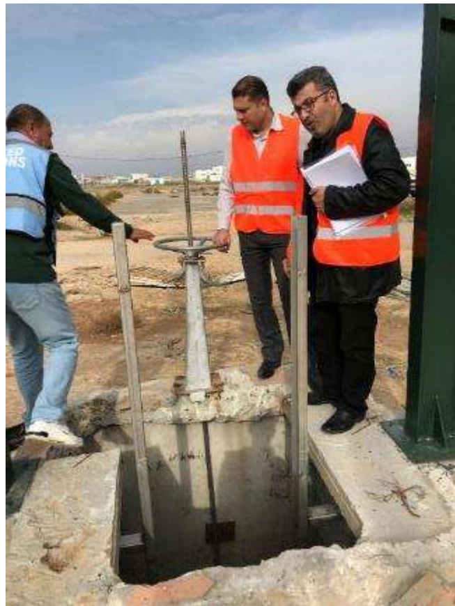
Fig. 13: Field Audit Team Evaluating the Sewage Pump Station
