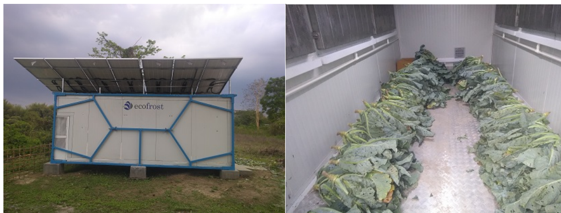
Outside and inside views of one of the six 5 ton solar PV cold storage units in Assam supported by the project with 100% grant. The project has supported two such units in each of the three demo states. Photo take in April 2019.
