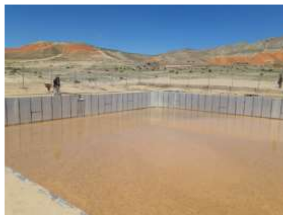
Figure 3: Sorkhoch and Mirji rain water storage, Balkh
