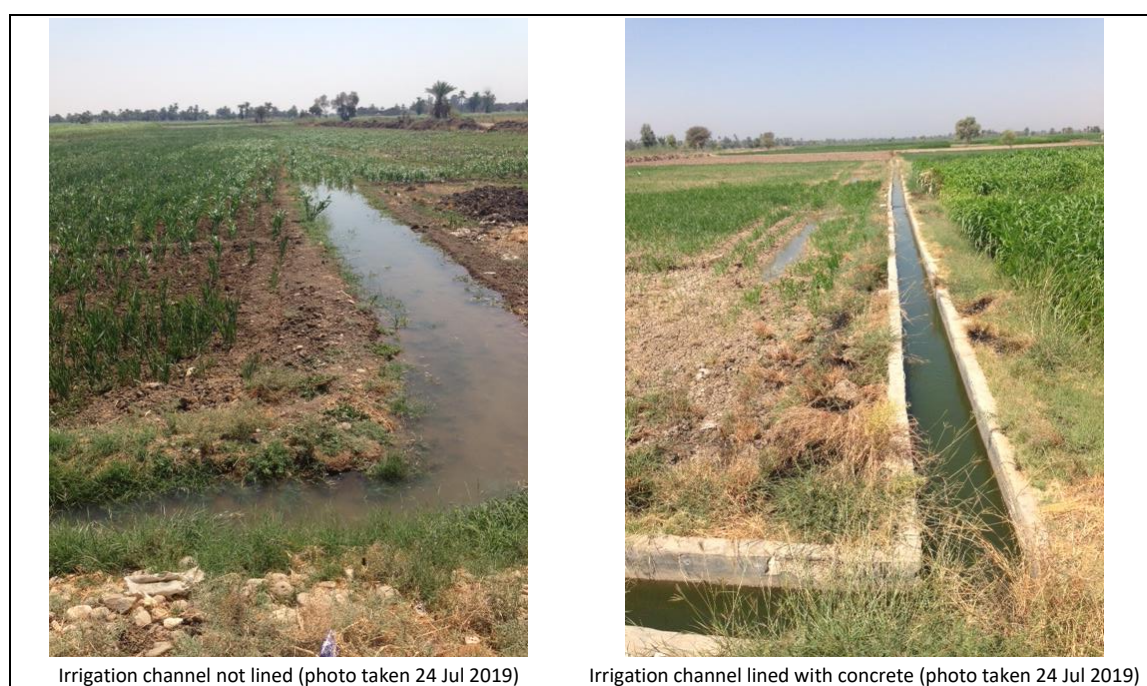
Figure 4: Irrigation channels lined with concrete under OP5, Qena Governorate
