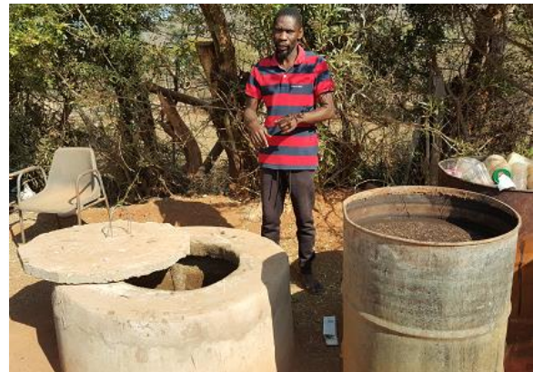
Household Biogas Digester in Otse village
