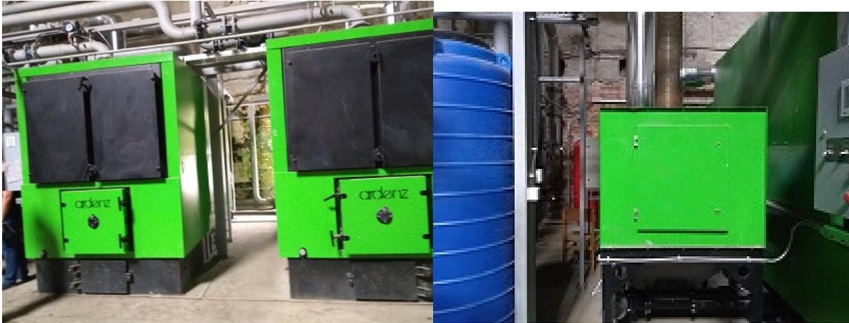
Left: Two of the three boilers of Odessa #11 Hospital 4.5 MW sunflower husk boiler system. Right: Feeder at Odessa #11 Hospital (holding the feedstock) for one of the boilers.
