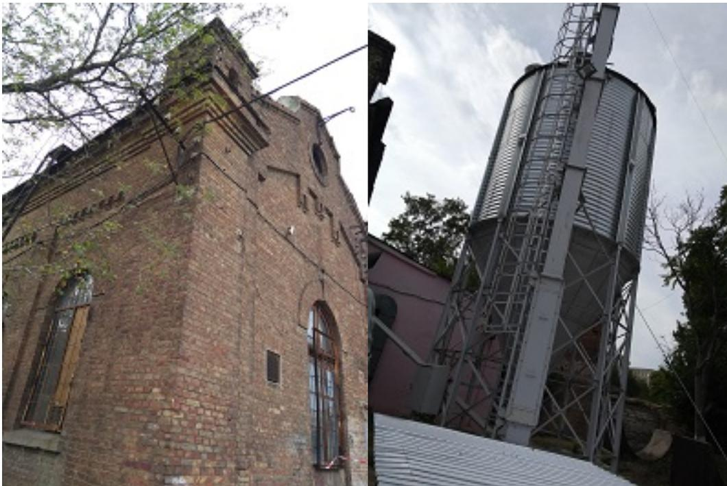
Left: Boiler house at No. 11 Hospital that is rented by private company for the biomass boilers. Right: Pellet tank, with cover of underground pellet storage area in the foreground. It's cheaper to dump pellets into underground storage and use a motor to lift them than to buy bagged pellets and have a crane to lift deliveries to high storage tank directly.
