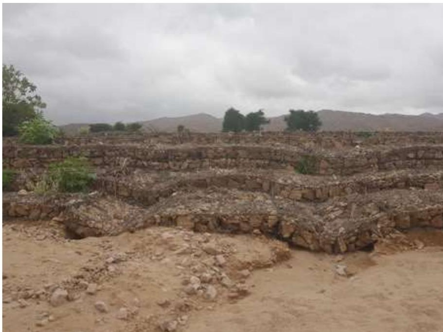
Picture 2. View from the upstream side of the Assamo micro-dam. The area where people are standing used to be 2 meters below the level of the micro-dam. Three years after its construction, sand and rocks carried by wadi waters filled this space, and the upstream wadi bed is now level with the micro-dam. Unless the height of the micro-dam is raised by adding another layer of gabions, it will soon be overflowed by sand and rocks.
