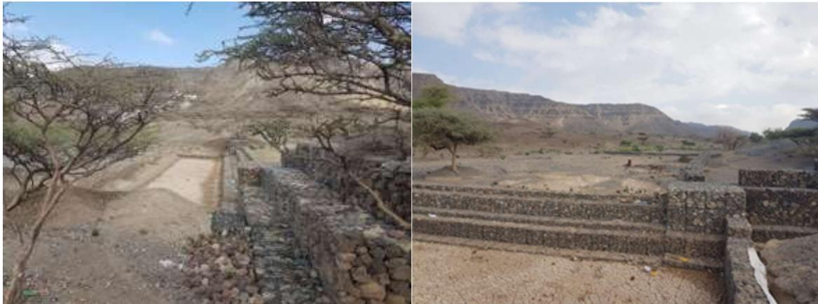
Pictures 4a & 4b. Two wells in the Adailou area. Located in or just next to the wadi beds, these wells are vulnerable to floods, that can damage them and pollute their water. The triangular structure on Picture 4a was built to protect this particular well from floods. Several wells were thus protected, each time taking the topography of the wadi bed into account to design the protections. Most existing wells were also further excavated.
