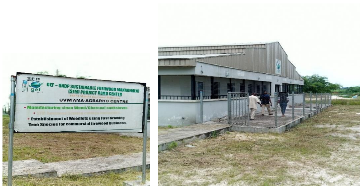
Photo 26 - Agbarho Multifunctional Platform (MFP) or Demonstration Centre
