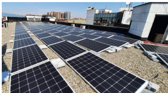
NAMA 1 and 2: Insolation of roof and installing the Solar PV
