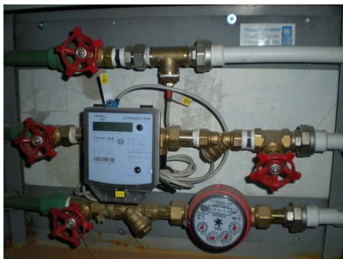
Heat meter installed at the entrance to an apartment in Avan district of Yerevan, as part of heating trials in 3 buildings
