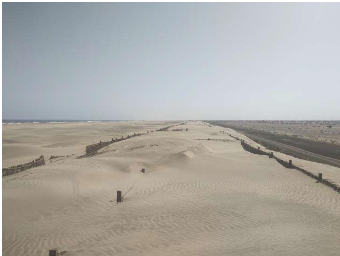
Figure 10: Option 2 illustrating condition of the dyke 4 years after construction
