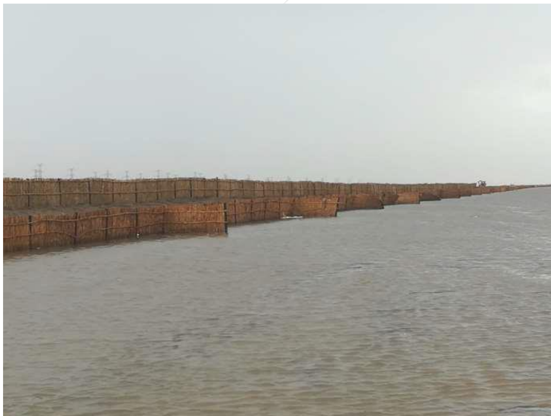
Figure 12: Flood reduction benefits of soft coastal protection structures in Kafr El-Sheikh
