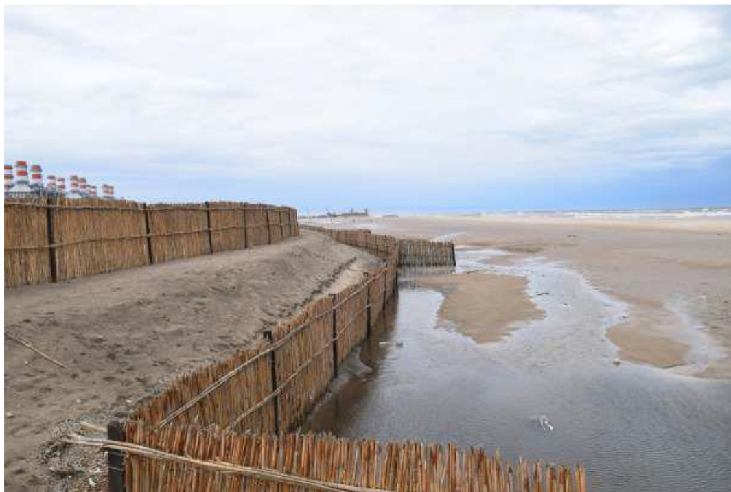
Figure 11: Flooding reduction benefits of soft coastal protection structures around Burullus Power Plant
