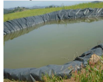
Plastic water reservoir
