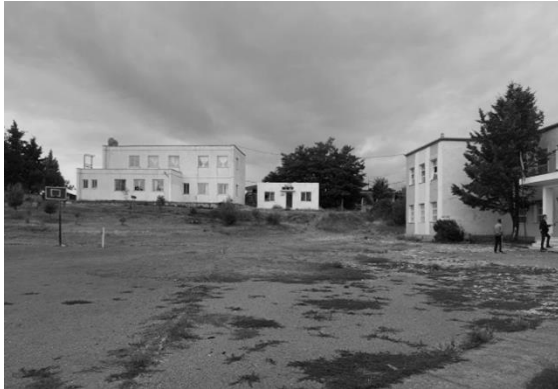
(4) "Ismet Nanushi" Joint School, Durrës (repair)
