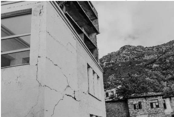
(20) "Skënderbeu" High school, Krujë (repair)
