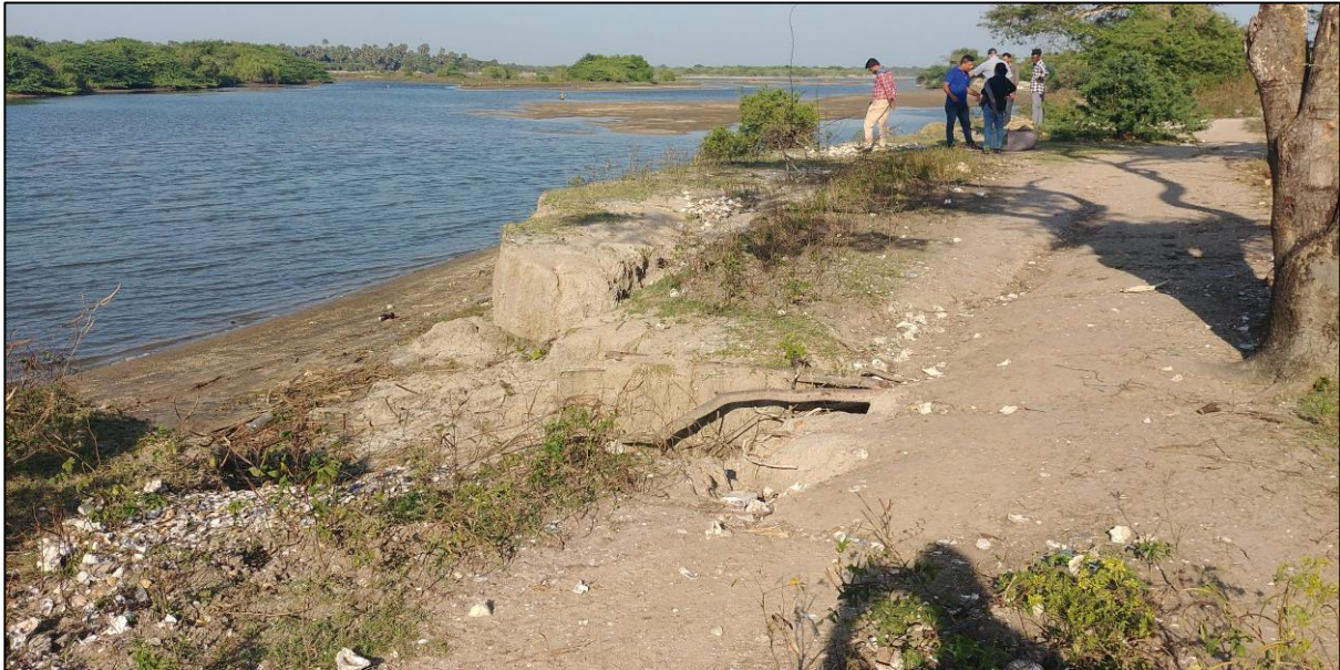
FIGURE 6: Example of coastal erosion and protection issues in TL3 – mouth of the Malwathu Oya River
