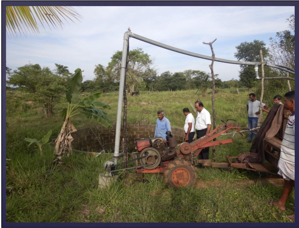
FIGURE 11: Any further agriculture activity that might be undertaken should focus on truly ecologically sustainable methods only – such as replacing diesel-powered irrigation pumps such as this one, with solar-pumps throughout all three TLs. This would be an extremely beneficial intervention, not only improving ecological sustainability, but also significantly reducing production costs by eliminating the need for farmer to purchase diesel
