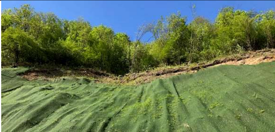
Senokos-Lomnica - site 1: Upper part of the net not fixed to the ground and regressive erosion above the net
