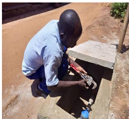
Photo: Akuei Malang Carrying out Plumbing
