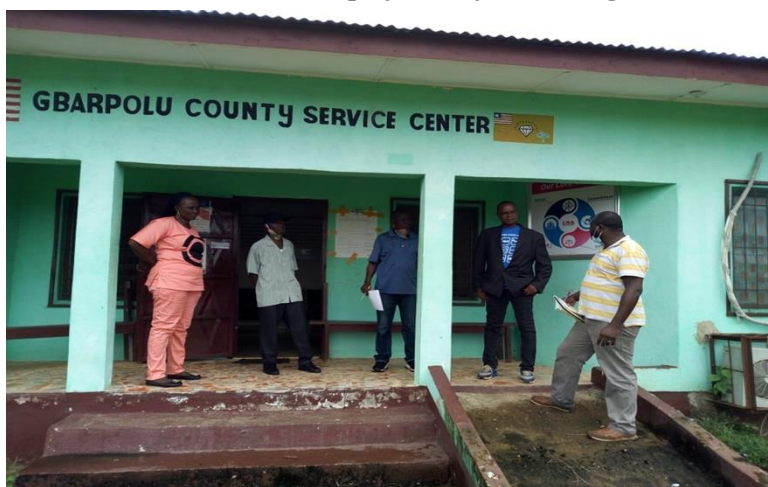
Ramp besides the steps to enable access of PWDs wheelchair users
