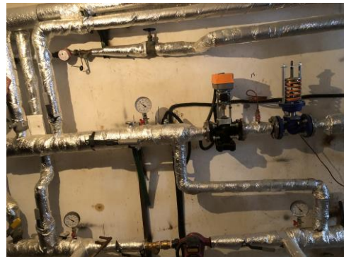
Heating system improvements
