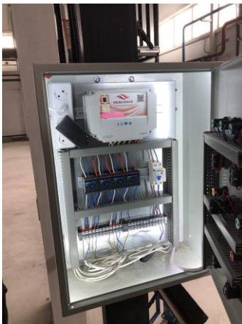
Chip board installation near heating station
