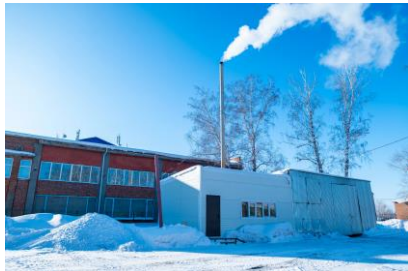
Biomass heating plant
