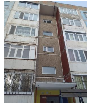
Apartments after improvements
