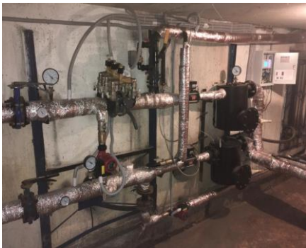
Heating system improvements
