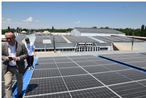
Solar array across plant roofs
