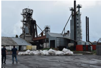
Biomass heating plant
