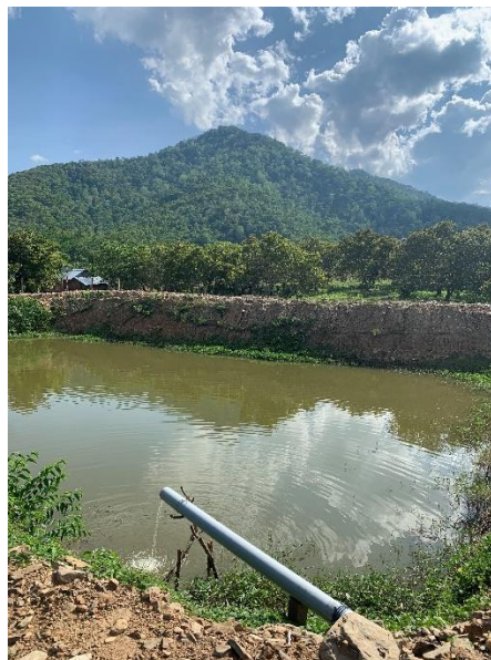
Photo 2. Typical pond construction: note steep sides
