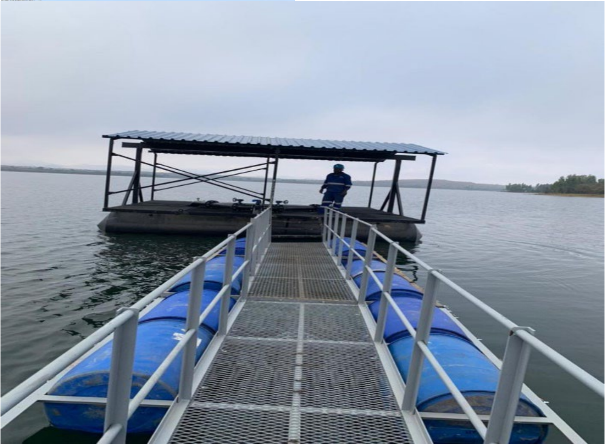
Figure 3: The civil works at Zvinyaningwe
