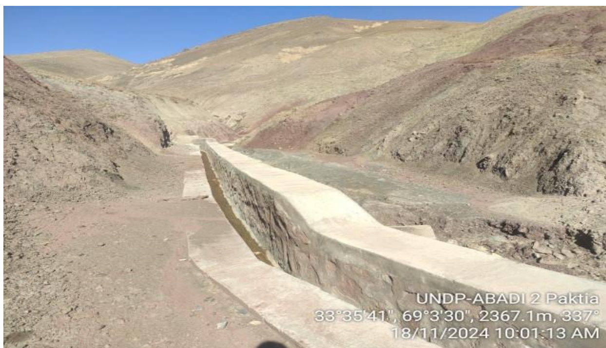
Figure 16: Protection wall in Paktia
