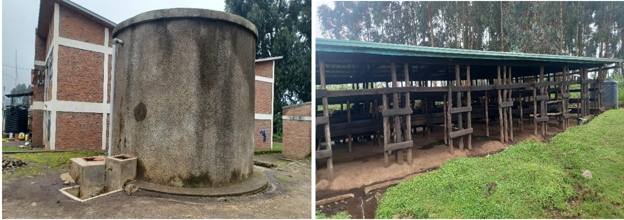
Water tank of 100m 3 (left) cow shed (right) in Mudende IDP village, Rubavu District
