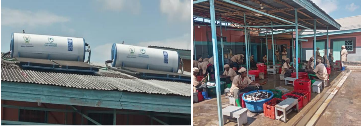
Solar water tanks (left) and bottle washing (right) at Buganza Good Wine, Kayonza District
