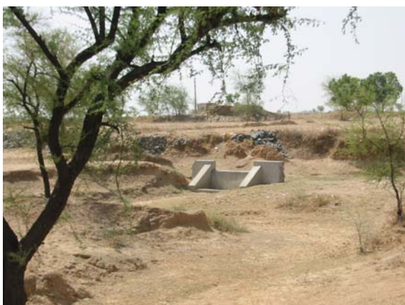
A drop Spillway
