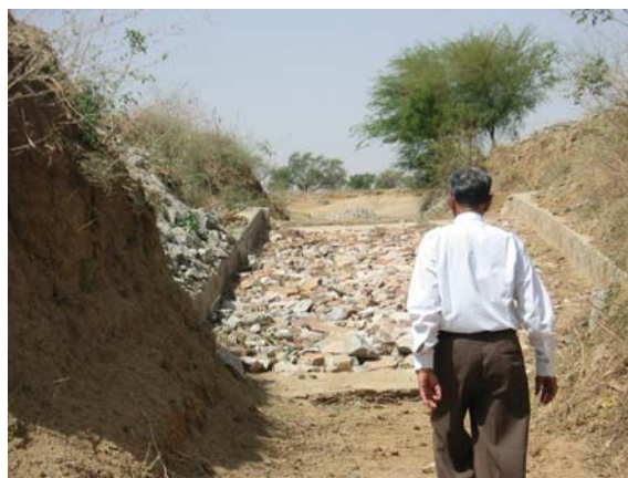
A Weir-cum-Ramp in the Cart
