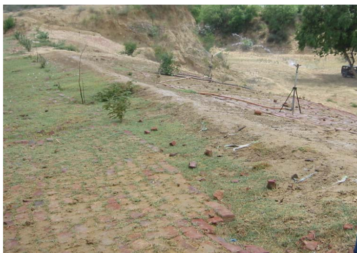
Pitching and watering at the check dam
