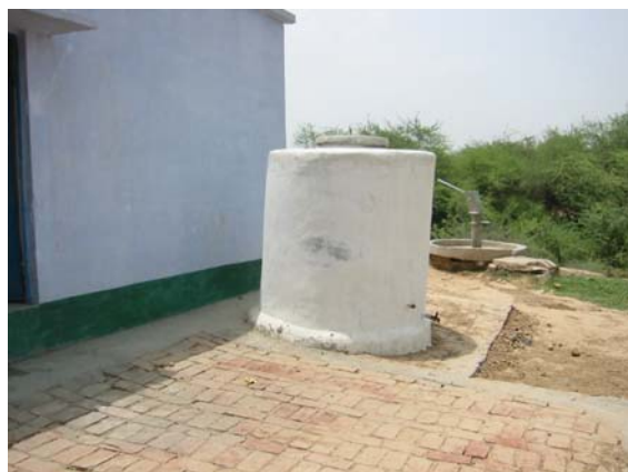
A Ferro-cement Tank in a School
