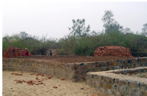
A tourist lodge constructed up to the plinth level
