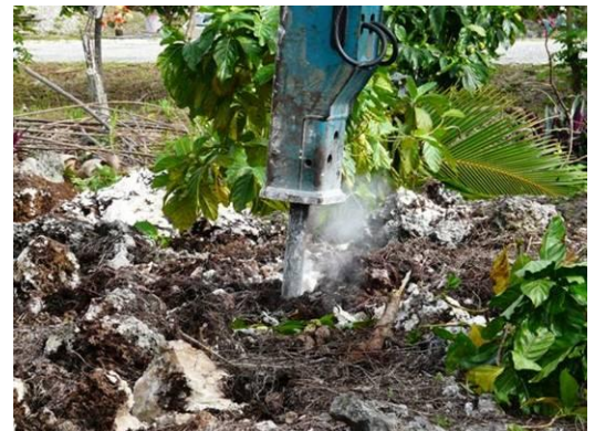
Photos: Rock breaking working within nonu plantings
