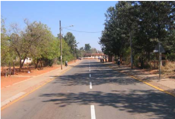
New sidewalk in residential area
