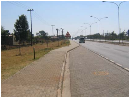
New sidewalk and bus/taxi stop
