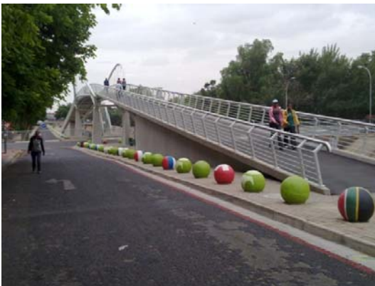
Selborne pedestrian bridge
