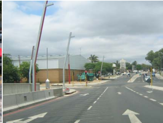
Upgraded signalised intersection with protected sidewalks on bridge
