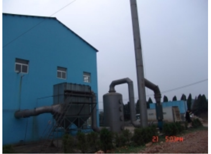
Photo 8 – Medical Waste Incinerator
