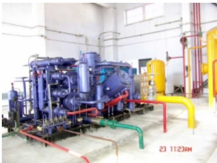
Photo 11 – High Pressure Compressor 2
