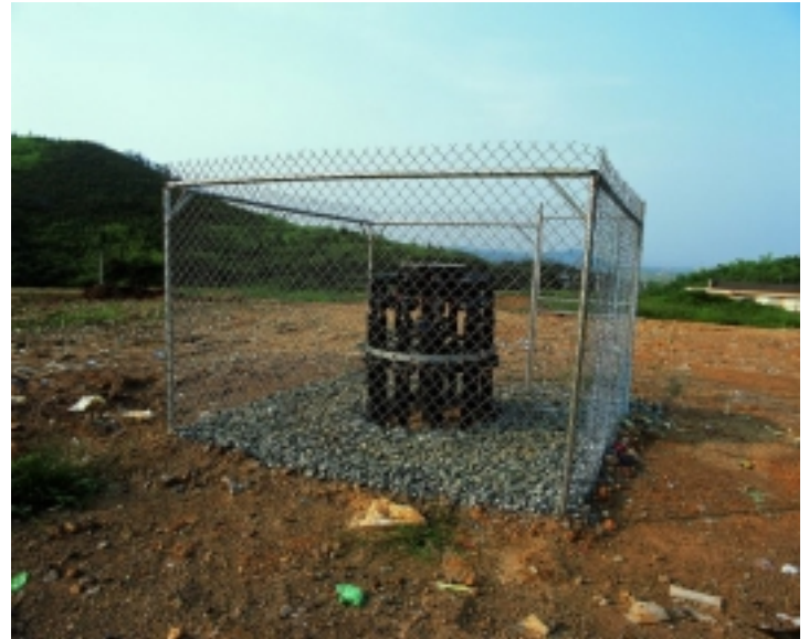
Photo 14 – Wellhead Cluster
