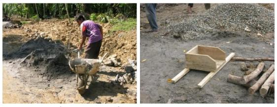
Fig. 8. Devices for measuring and transporting
