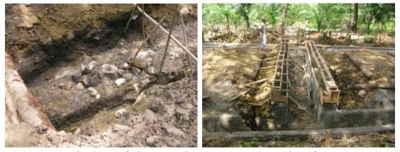
Fig. 10. Foundation work for Box Culvert Fig. 11. Steel work
