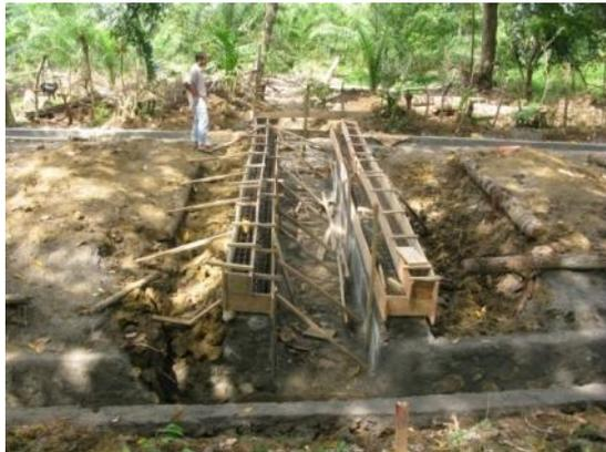
Fig. 10. Foundation work for Box Culvert
