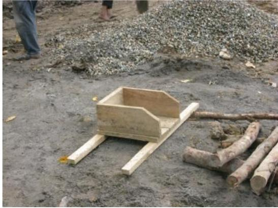
Fig. 8. Devices for measuring and transporting
