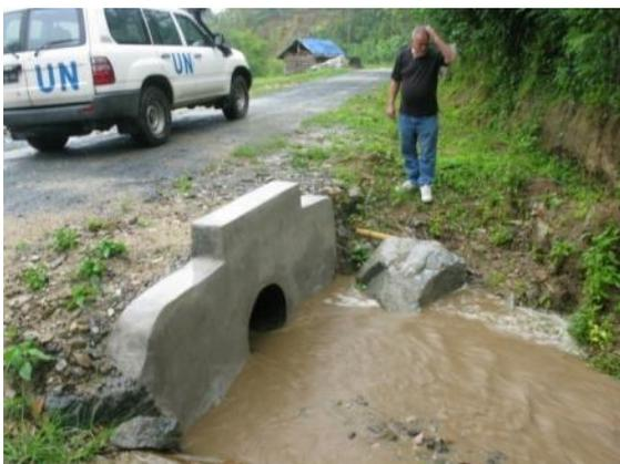
Fig. 3. Box culvert section
