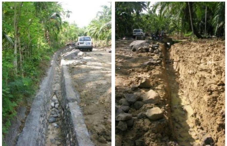
Fig. 7. Drainage works with stone masonry
