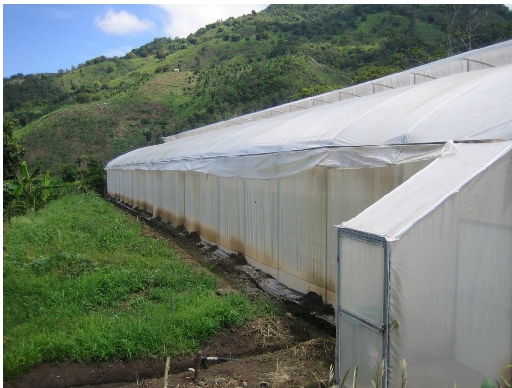
Figure 12 - Greenhouse for Intensive Agriculture Receiving Financial Support through the Project
