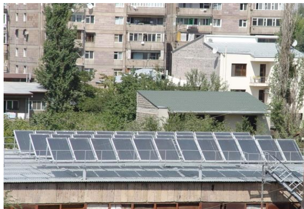
Figure 5.1. Solar water heaters, Avetisyan street energy centre
