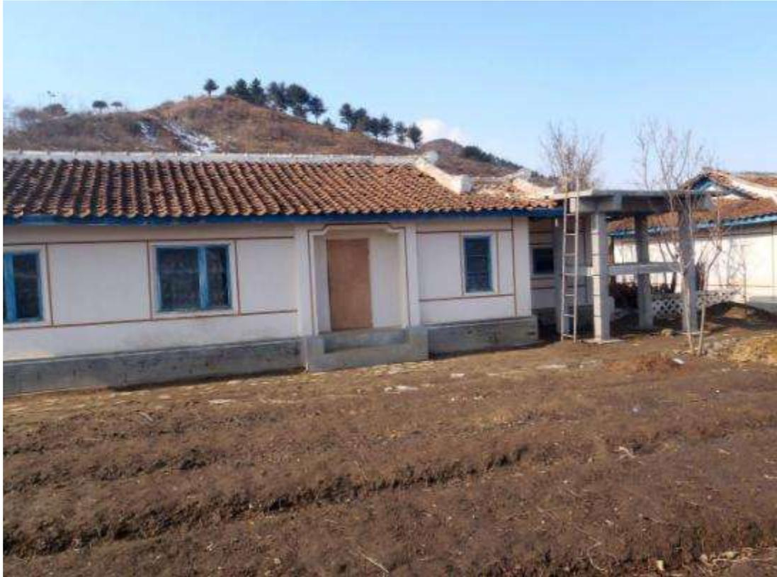
At Mopung, thermal isolation for houses will be provided, as well as solar water heaters. The concrete support for the SWH was in place, the systems are not yet delivered. Please note that low-temperature concrete is not easily obtained in DPRK; by consequence, activities are suspended in winter time. Also here, the SWH support structure dims the light at the nearby window.
