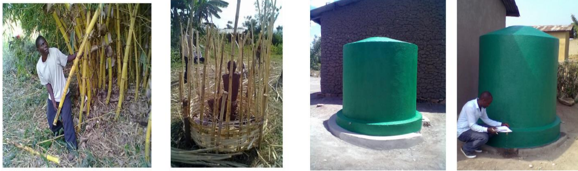
Photo: The water tanks are made of Bamboo, sand and cement
