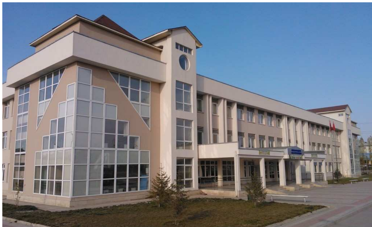
Picture 1: First energy efficient pilot school in Kyrgyzstan, School No. 52 in Osh
