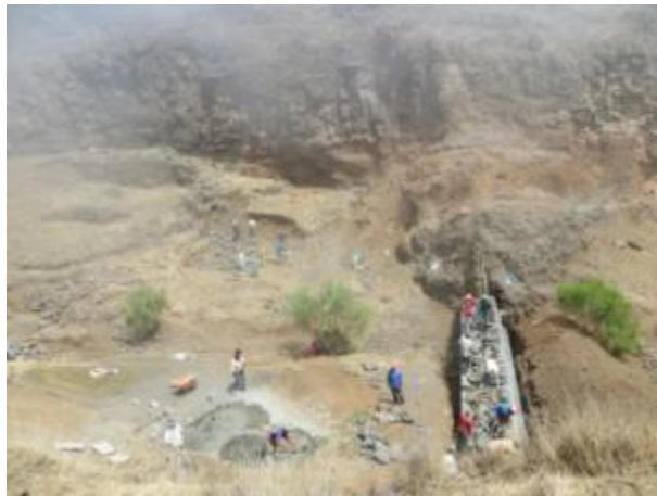
Pictures 2 & 3: Check dams contributing to ground water recharge in Ribeira Grande upper catchment
