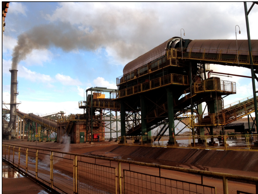
Figure 3. Trash cleaning system and chipper, Usina Alta Mogiana, 2013
