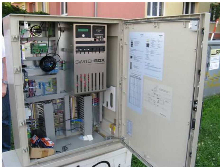
Figure 3: Tram signal priority equipment installed at the Pekna Cesta intersection along the Racianska Corridor
