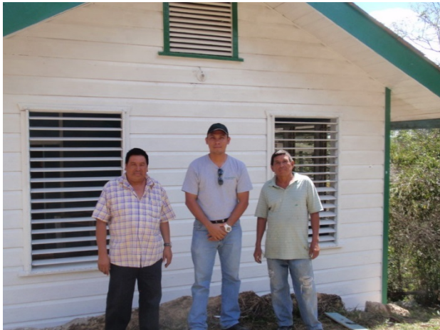
Refurbished Staff Quarters, Mountain Pine Ridge Forest Reserve, 14 Mar 2015
