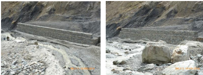
Gabion Protection walls at Gobashedeh (Drongagh).
