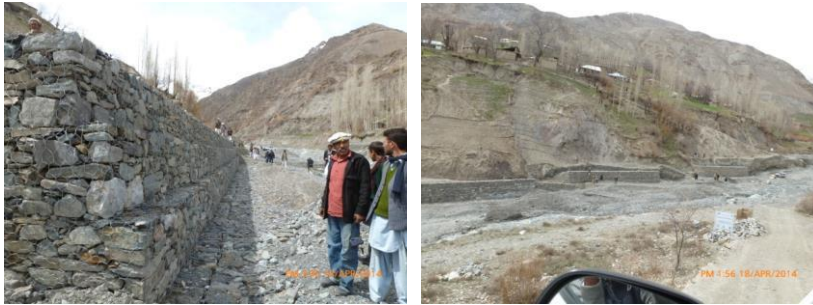
Gabion protection walls at Bindo Rathani (Drongagh)
