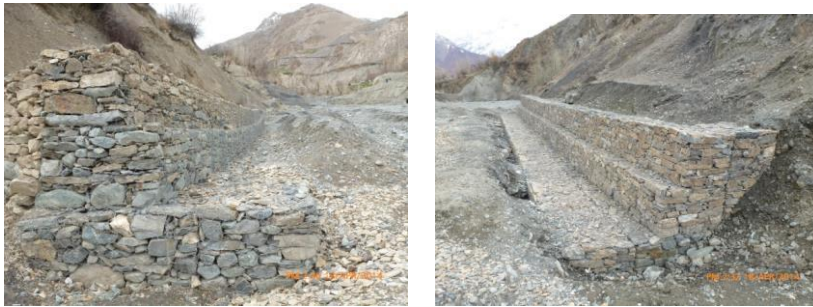
Gabion protection walls at Pongodur (Drongagh)
