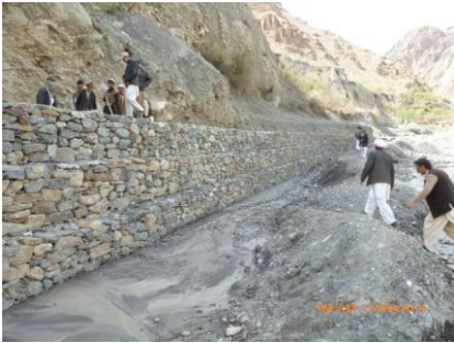
Gabion protection walls at Shogram village
