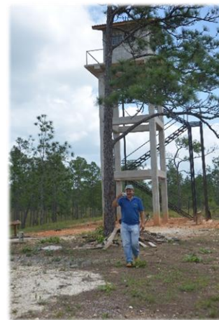
Figure 3: Fire observation tower built with CLIFOR funds near Mabita.
