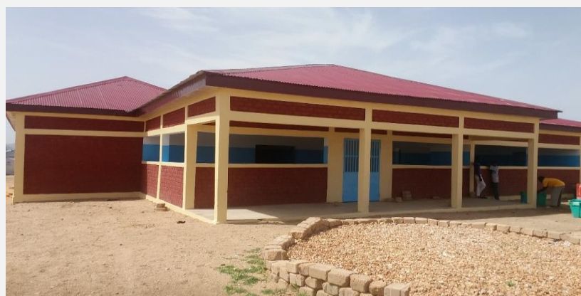
The completed health centre built by Mr. Djagra's social enterprise using stabilized soil bricks (SSBs)
