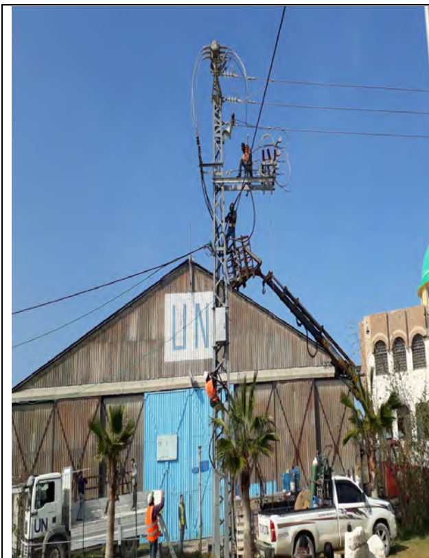
Connecting the lighting network to the main electricity network
