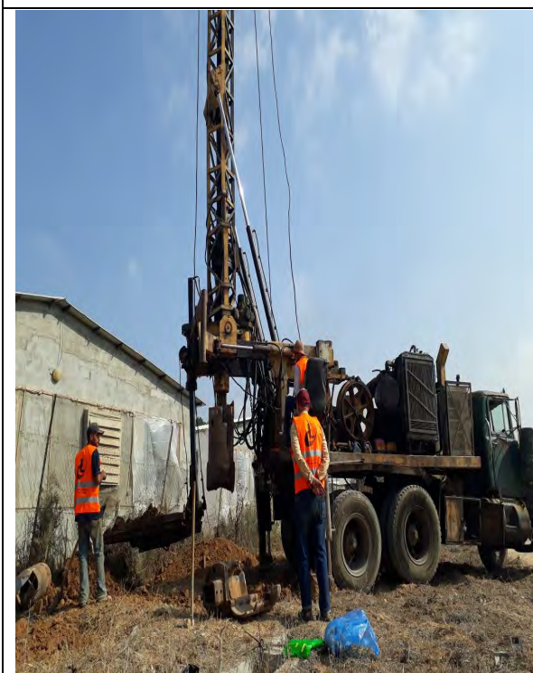
Drilling works of the new water well
