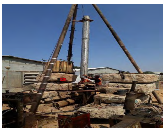
Drilling works of the new water well
