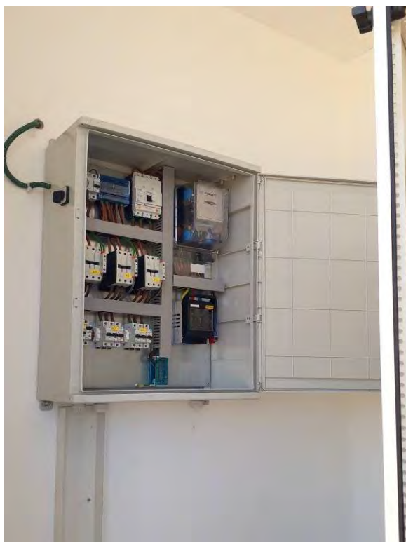
Installation of lighting control panel box
